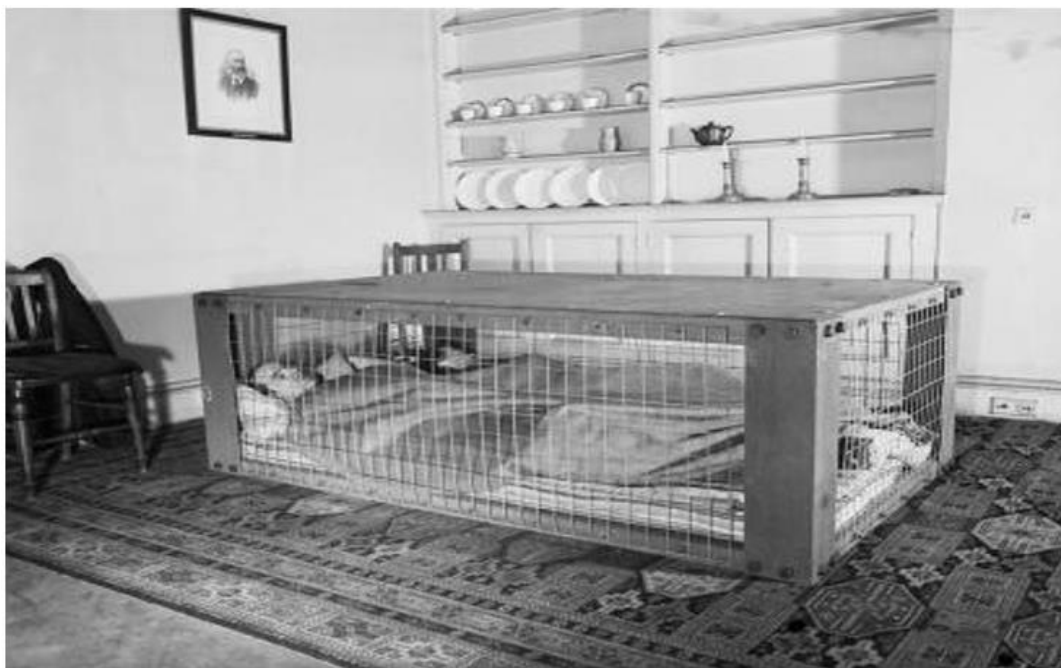
Figure 3. Morrison air defense shelter in use.
