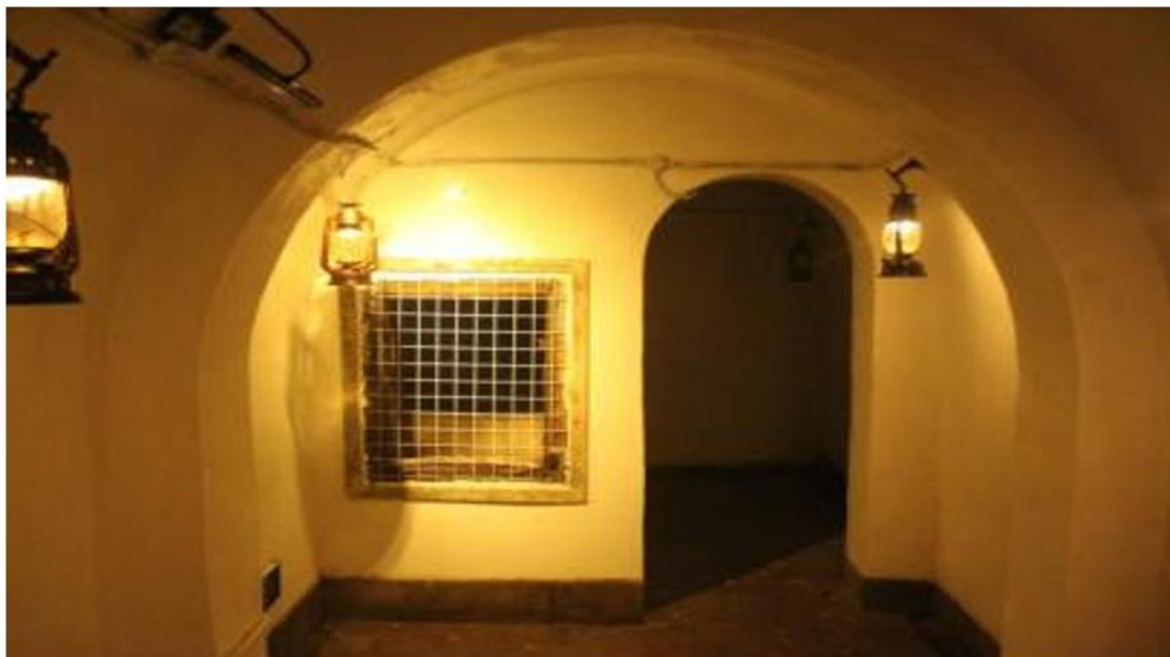
Figure 5. Internal food elevator in the Yiyuan.
